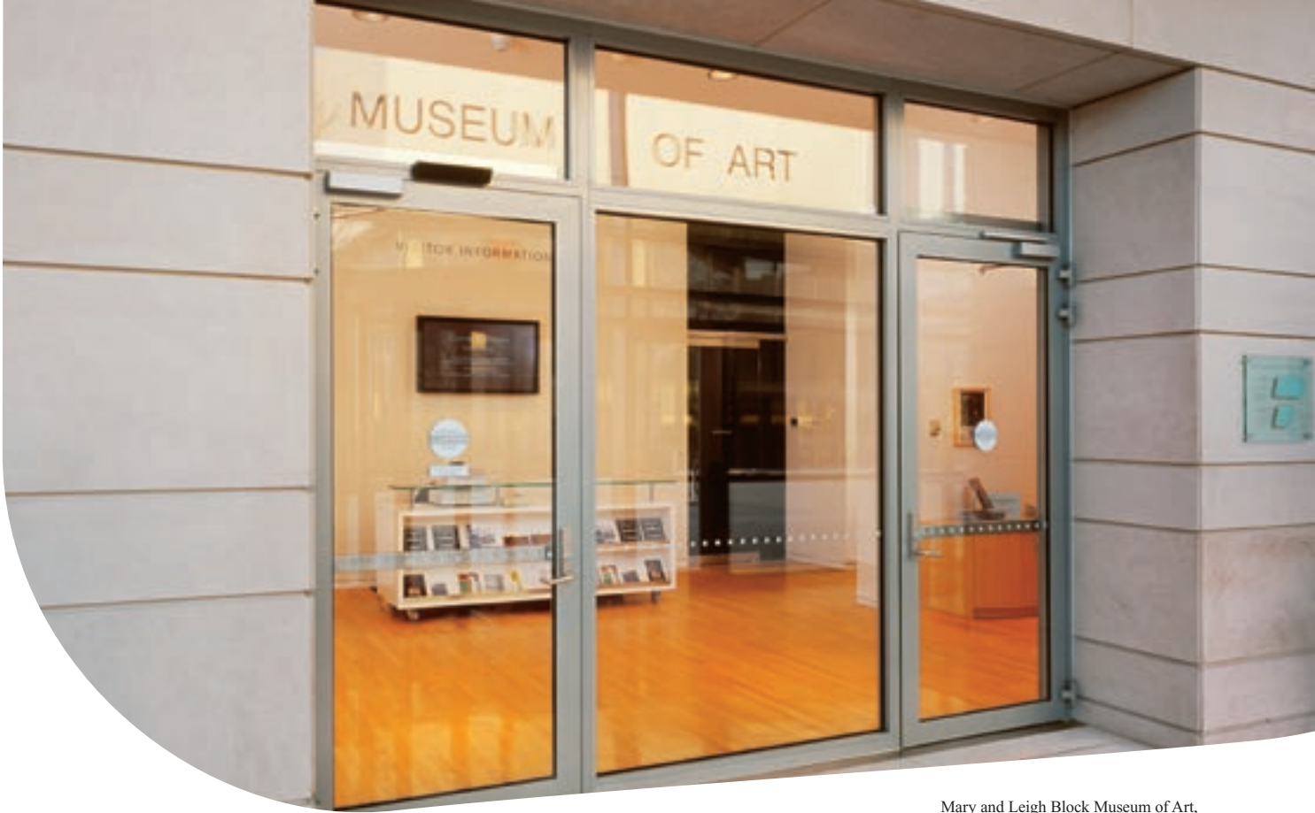
Mary and Leigh Block Museum of Art, Evanston, IL: Partition with doors glazed with Pilkington Pyrostop™ secures safe escape in case of a fire.
