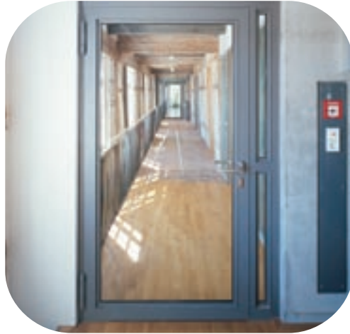
– Image left – L'Anse Creuse High School, Harrison, MI: Partition with a double leaf door glazed with Pilkington Pyrostop ™ .
